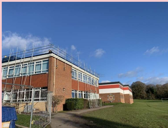
Scaffolding has become a familiar sight
